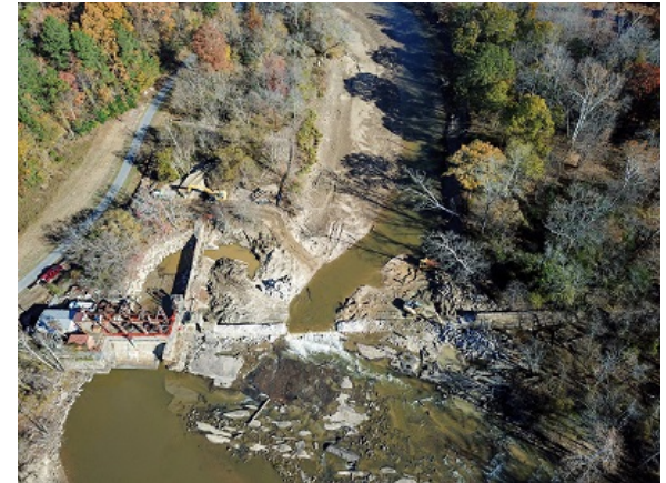
Milburnie Dam Removal, Nov. 2017
