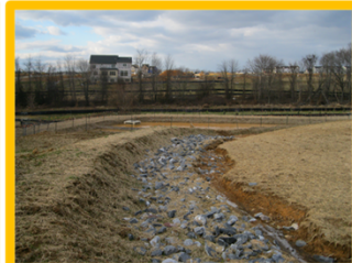
Land grading with erosion and sediment control
