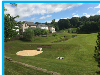
Suburban with green stormwater infrastructure
